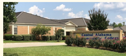
Childersburg Campus 34091 US Hwy 280, Childersburg, AL
